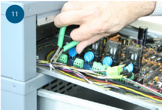
11 Cut wire ties on left side wire harnesses
