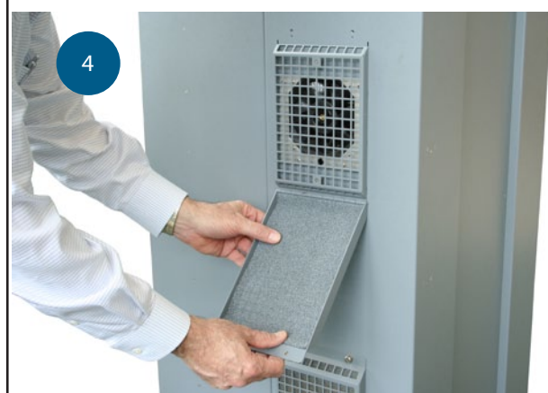
4 Hinge up Tighten thumbscrews
